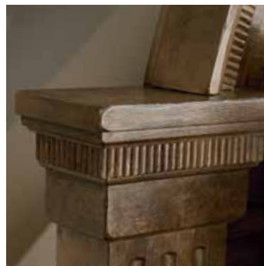
Old brick walls which surround Kentucky horse farms and pastures inspired the stair-step post design and dentil molding.
